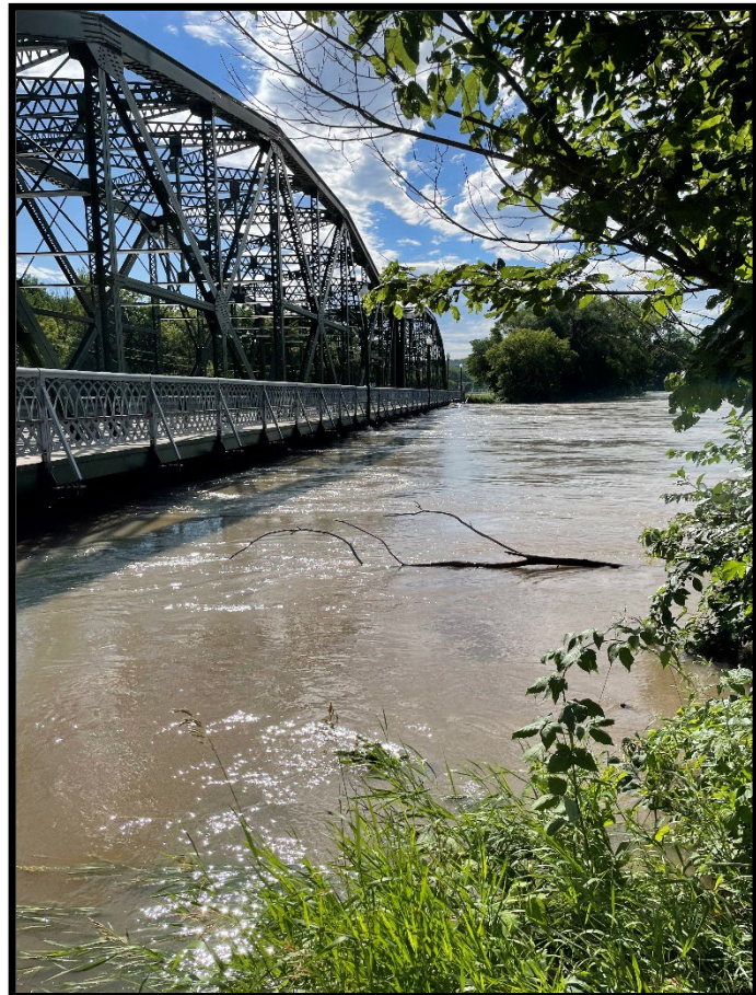
Figure 13. Hwy 99 Bridge in Saint Peter, MN. Photo Credit: Holly Bushman
