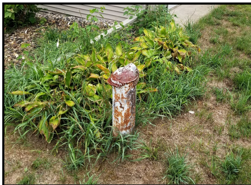
Figure 2. Residential Well on Lake Shore Property. Photo Credit: Holly Bushman.
