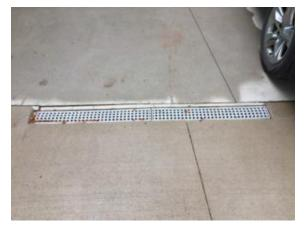
The steep driveway created a challenge especially in the spring with frost still in the ground and a slippery, sloppy, muddy thawed layer on top. It was a perfect recipe for gully washes with spring rains. The solution was constructing a small paved driveway with a drain underground.
